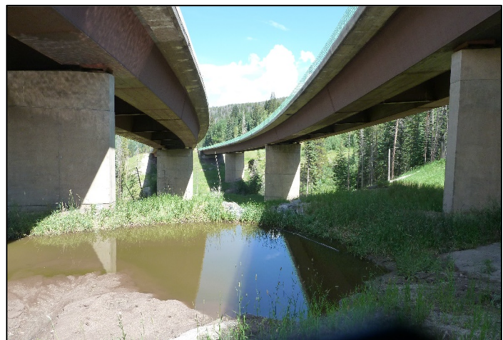
Figure 6. Bridge at MP 185.2 Allows Unimpeded Wildlife Movement Through the Highway Corridor
