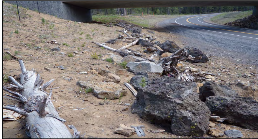
Figure 19. Wildlife Lane Incorporated into an Existing Underpass Originally for Vehicle Use Only. Logs and Boulders Were Added to Promote Wildlife Use. Source: Ruediger and Jacobson 2013.
